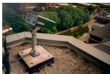
100Mbps Data link installed for major financial institution, connecting remote offices in Reading, UK. Installed 1998.
