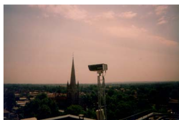
CableFree unit on 2m tower mount to create line-of-sight for a 100Mbps LAN-LAN extension link over 1.2km. Installed UK 1996
